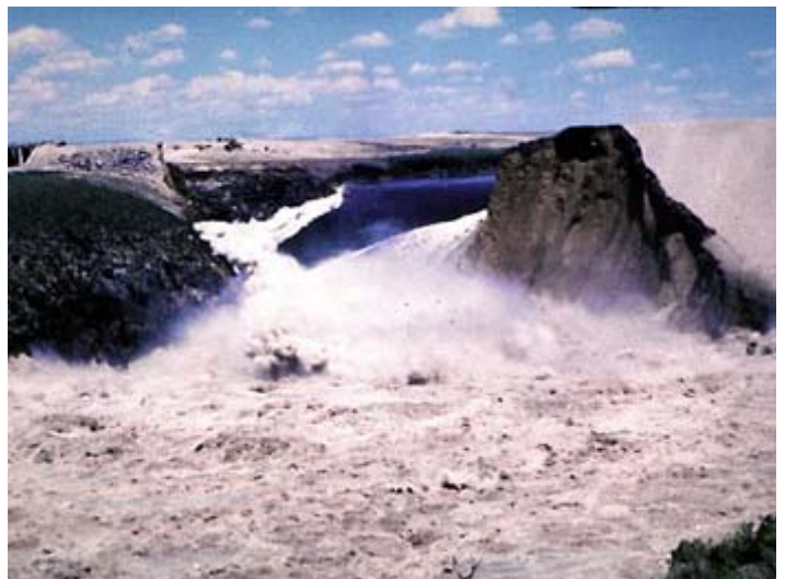
Teton Dam Breached, June 5, 1976
